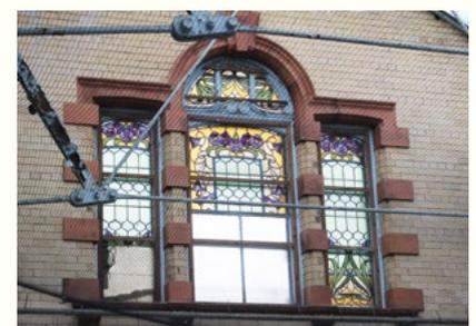
Photo: Females Pool North Window in a very poor state of repair, this work will return them to their former glory and keep the rain and wind out.
